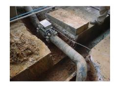
PORCUPINE - Internal Defect Mapping
